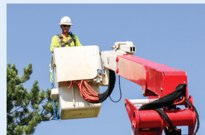
Eddie Ruiz removes tangled wires caused by high winds.
