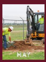
Linemen work to reroute overhead lines underground at Roundup Arena.
