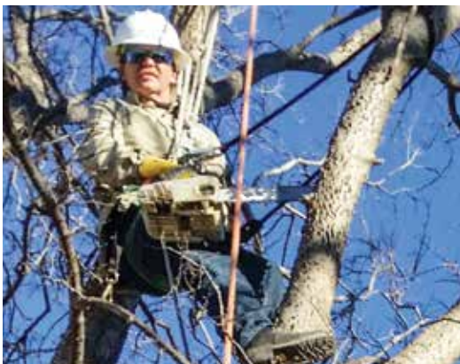
Steve Jimmerson trims limbs away from a power line.
