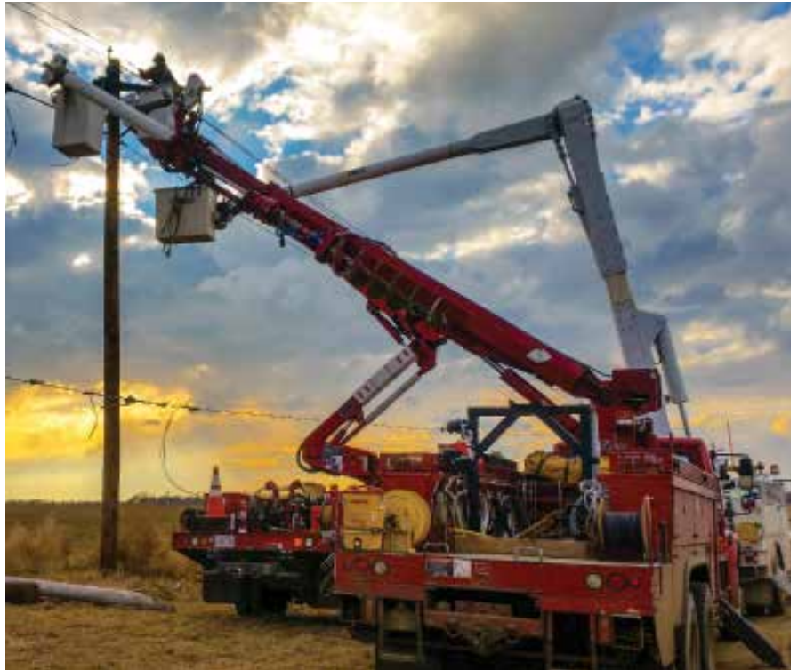
Victory Electric crew restores power during the January 2017 ice storm.
