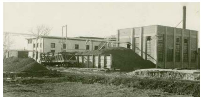
The boiler house and coal plant. During the ice season, 34 tons of pure crystal ice were manufactured daily in the building in the left background.
