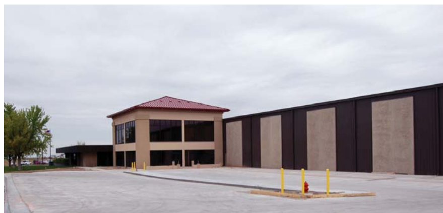
On May 4, Victory's 37,000 square-foot expansion was complete.
