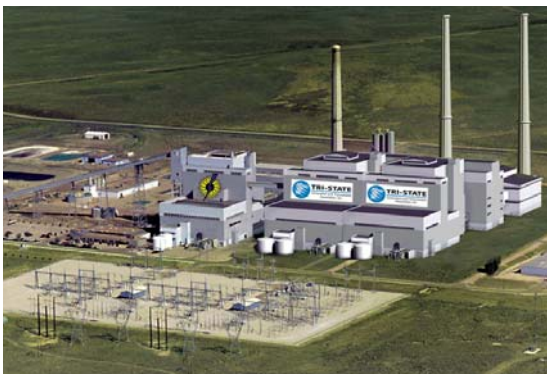
Above is the original proposal for the Holcomb expansion, which included 1,400 MW. The compromise will result in the elimination of one proposed unit and net 895 MW.
