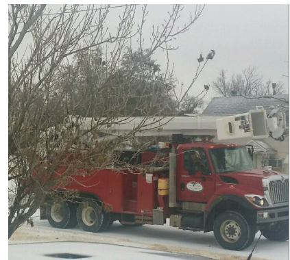
Victory crews worked several hours during the ice storm until power was restored. Photo courtesy of Shelia Breensing.
