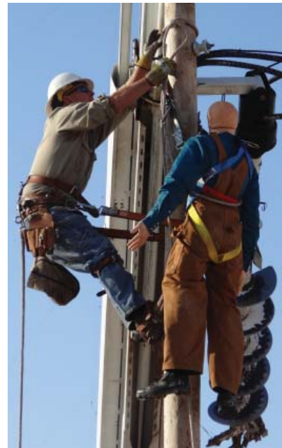
Dave Masden rescues a training dummy from the top of a electric pole.
