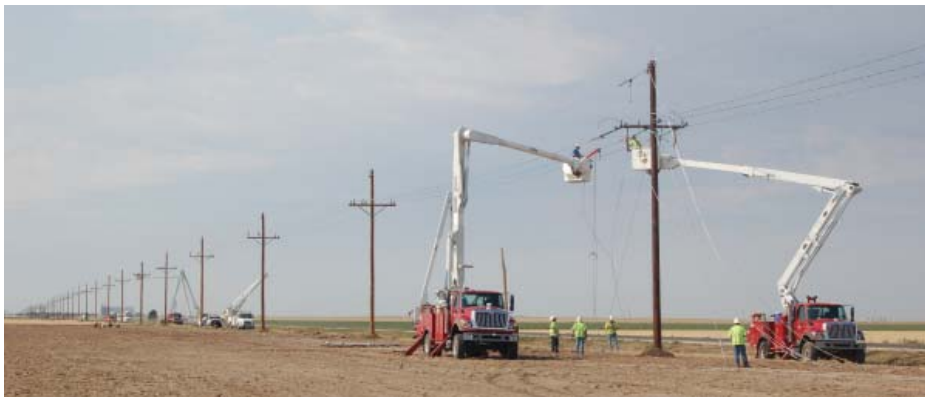
Left: Because of the extensive damage to the transmission line north of Minneola, Victory Electric elected to replace all of the existing structures and replace with new poles and wire. Victory crews spent the week replacing approximately three miles, or 80 poles, and restrung new wire. Right: The storm heavily damaged the Bloom substation.
