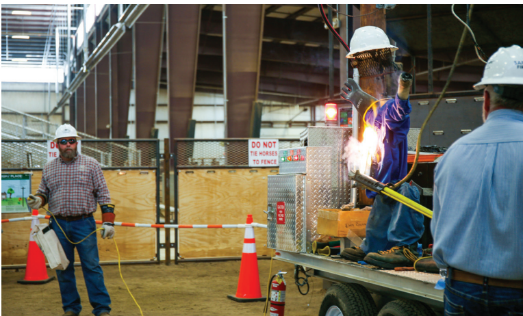
Mikey Goddard, vice president of safety, discusses the importance of safety around high voltage power lines.
