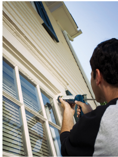
Sealing air leaks in your home can save you energy and money—up to $212 a year!
