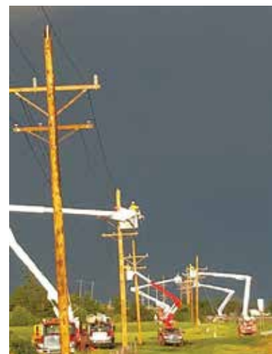
Lineman Jacob Ledford snaps a quick photo of crews working together to replace 3/4 mile of downed line west of Dodge City.
