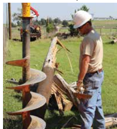
Lineman Clayton Stein replaces a snapped pole after the storms.
