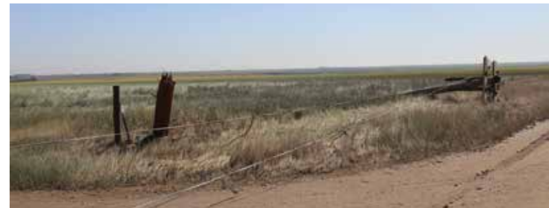
Downed lines and poles north of Dodge City caused days of work for crews.
