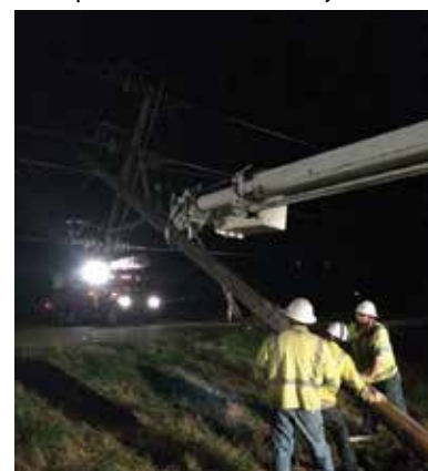
Crews continue to work and set a new pole the night of May 26.
